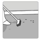
Ensure the sub floor is structurally sound. The sub floor should be clean and dry.
